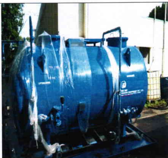
Fig.7: PCB contaminated oil stored in 6kl MS tank
