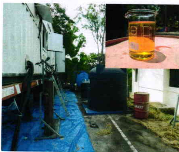
Fig.12: Oil after PCB de-chlorination stored in 5Kl Plastic tank for disposal
