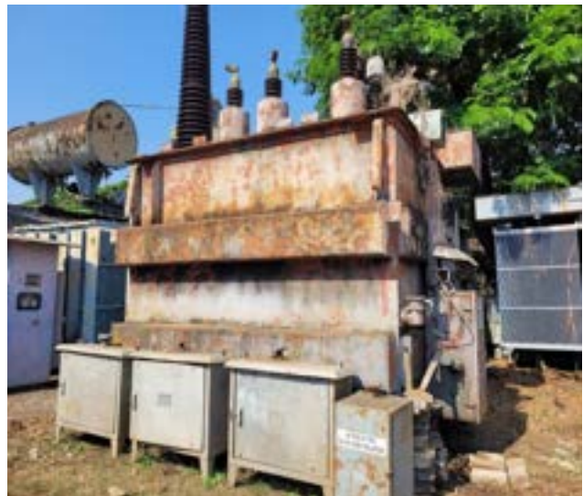
Figure 3&4: PCB contaminated 220/110kV GE Make Single-Phase Transformers @ 220kV Substation Nallalam
