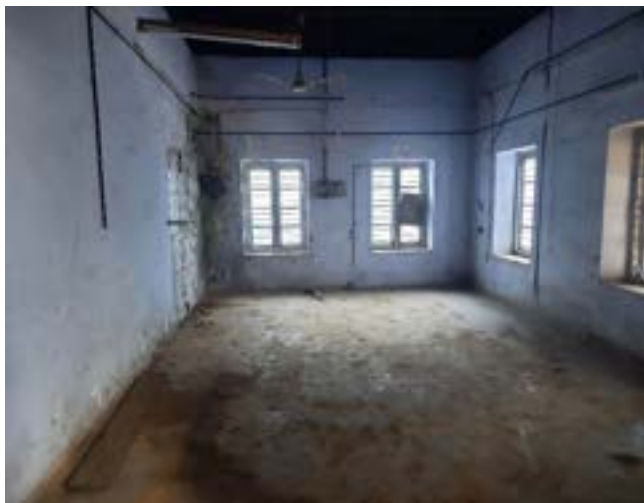
Figure 9: Storage room for storing PCB accessories.
