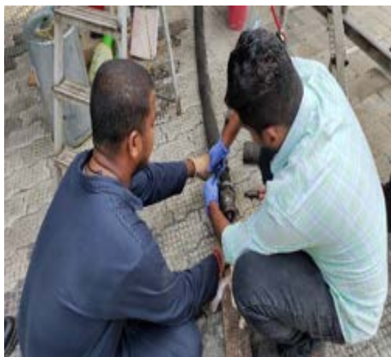
Figure 34: Fixing of outlet pipe for Unloading the dechlorinated oil
