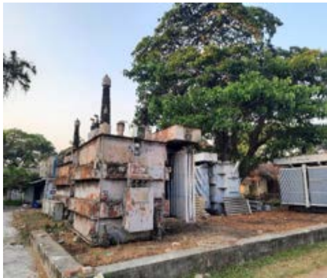
Figure 3&4: PCB contaminated 220/110kV GE Make Single-Phase Transformers @ 220kV Substation Nallalam
