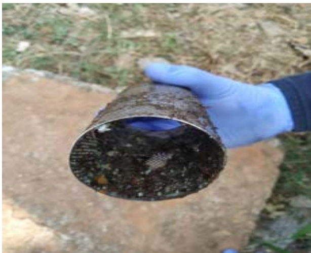
Figure 32: Chocked suction strainer
