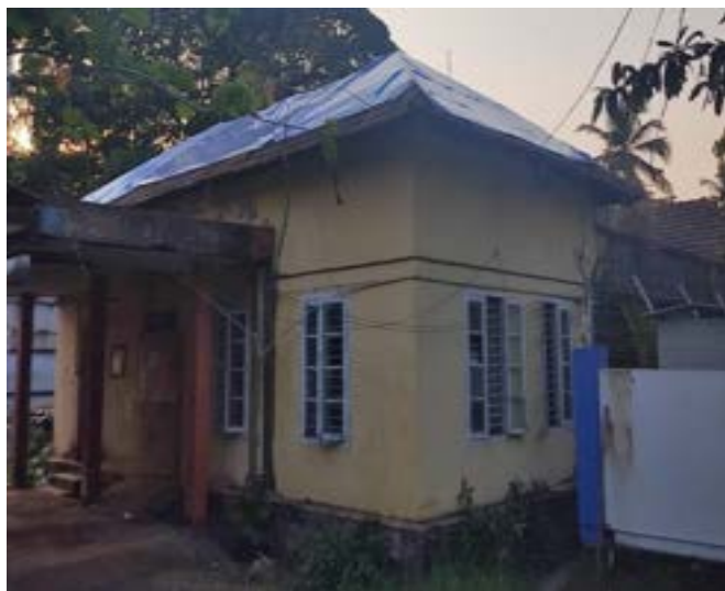
Figure 5: PCB accessories storage Room was covered with tarpaulin sheet.
