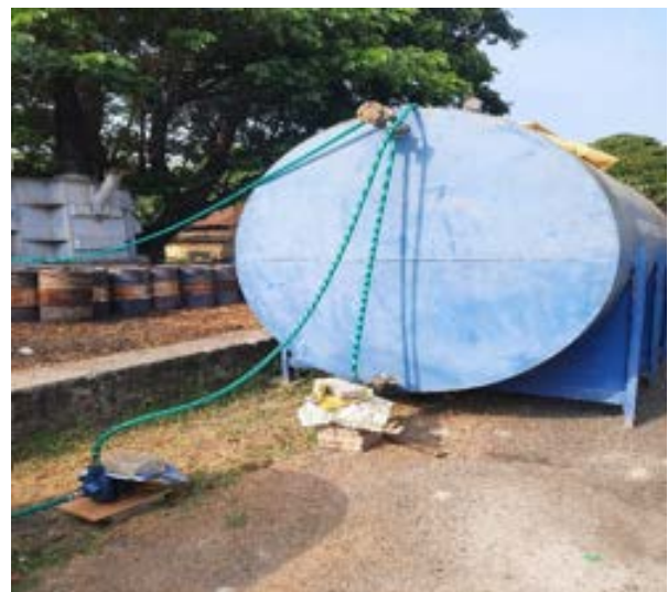
Figure 6: 15KL tank for unloading of treated oil kept near the PCB unit.
