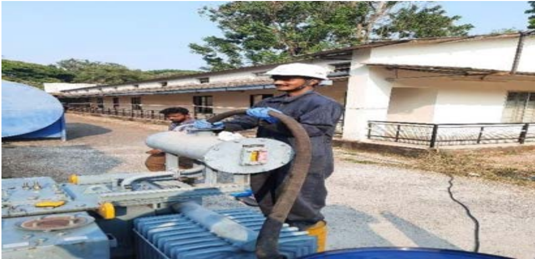
Figure 21: The step down transformer filling with fresh new oil
