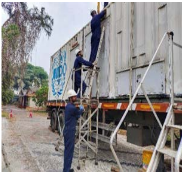
Figure 16: Fixing of exhaust vent to PCB unit.
