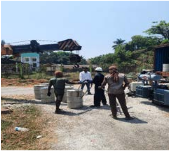
Figure 11: Unloading of sodium dispersion drums
