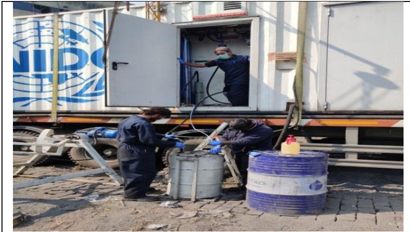
Fig. 5: Loading of Sodium dispersed oil (NaD) to storage tank
