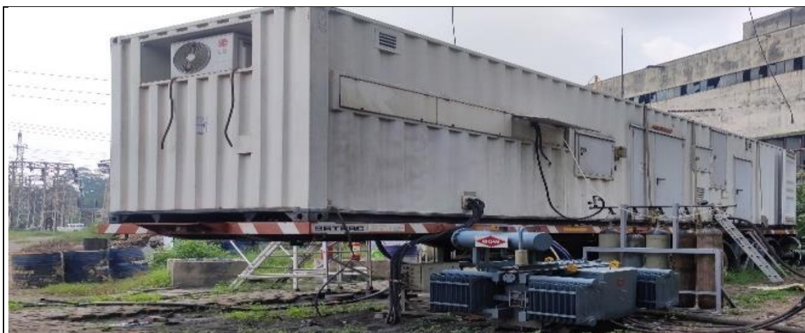
Fig. 3 : Placement of PCB mobile de-chlorination unit
