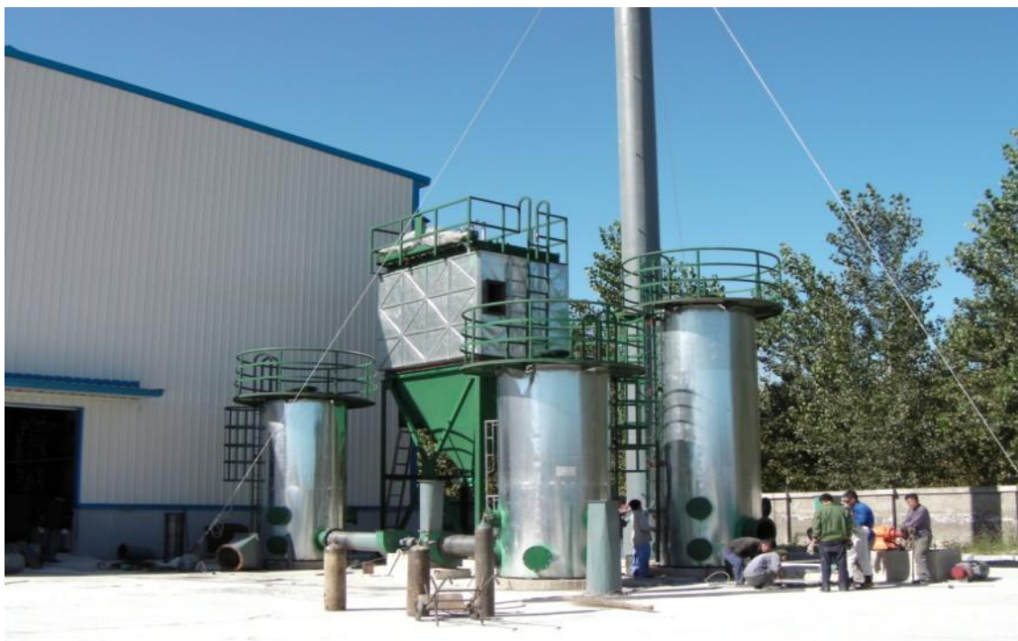
Figure 2 – An air pollution control system treating the emission generated by a PCB waste storage.
