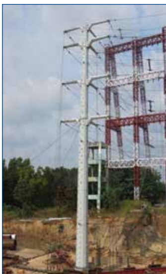
132 kV Multi Circuit Tower
