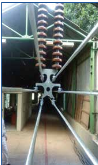
765kV HVDC Six bundle conductor
