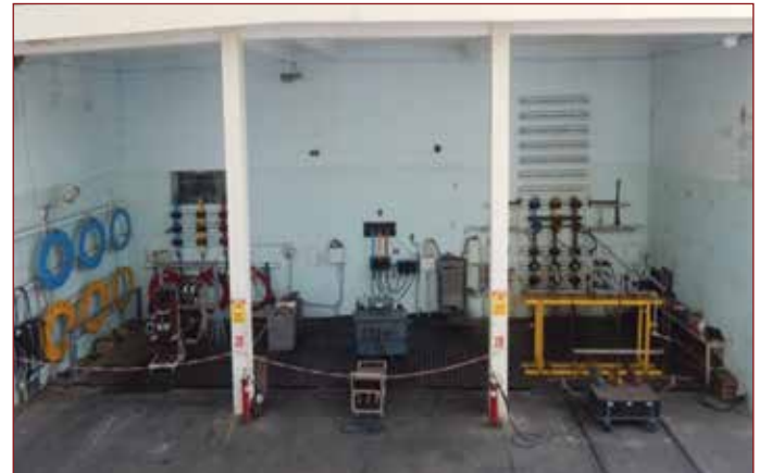
Short-Circuit Test Bays
