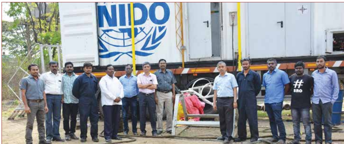
PCB Dechlorination work at VISL, Bhadravathi, Karnataka
