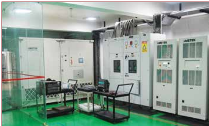
Grid tied Inverter test facility
