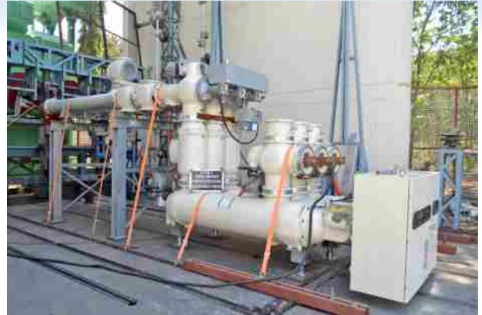
Short-time withstand current test on 245 kV, 3150 A, 50 kA GIS for M/s. Siemens Ltd., Aurangabad, Maharashtra
