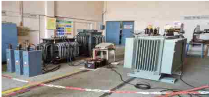
Temperature rise test, Sound Level measurement in no load & full load conditions were conducted on the transformer of M/s SGB Malaysia Compact substation as per cl. 6.1, 6.5 of IEC 62271-202, 2014. The tests were conducted in STL, CPRI, Bhopal.
