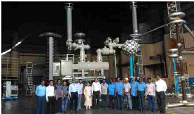
Visit of Kang dong wan, Lee Jongmin, Yun Jinwon for Dielectric and RIV tests carried out as per IEC 62271-203 on M/s. Hyosung T&D India Pvt. Ltd., Pune, make 420kV Gas Insulated Switchgear comprising of Circuit breaker and Disconnecting switches carried out at High Voltage Division, CPRI, Bangalore.
