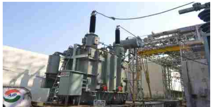
Ability to withstand the dynamic effects of Short circuit test on 21.6 MVA, 132 kV/27 kV Single Phase Transformer for M/s. Vishvas Power Engineering Services Pvt. Ltd., Nagpur
