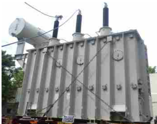
Ability to withstand the dynamic effects of short circuit test on 80/120MVA,132/33kV, Three Phase Transformer carried out at High Power Laboratory, CPRI, Bangalore
