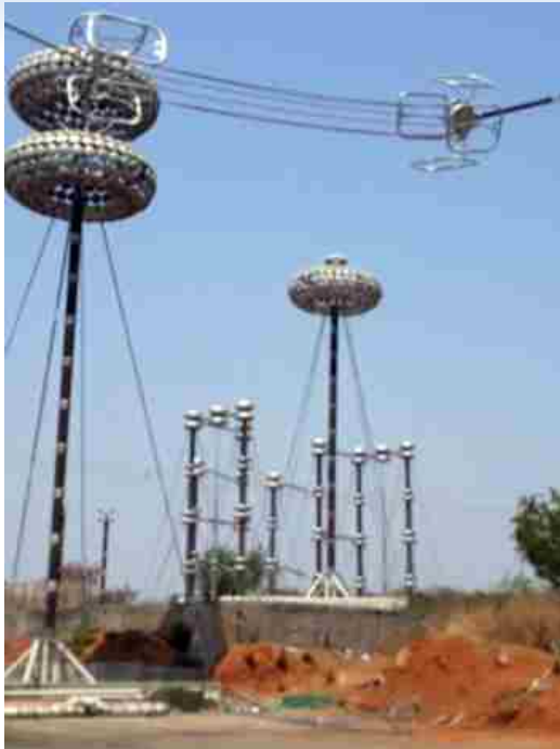
DC corona test on \pm 800 kV HVDC ACSR Hexagonal Lapwing Conductor Bundle for M/s. Neccan Power & Infra Ltd., Jaipur
