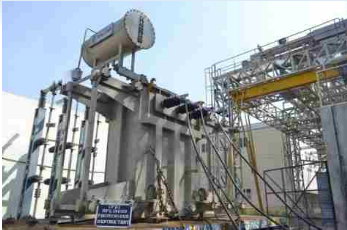
Ability to withstand the Dynamic Effects of Short Circuit test on 5 MVA, 33 kV/0.360-0.360 kV, Three Phase Transformer for M/s. Shilchar Technologies Limited, Vadodara
