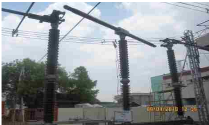
Short time withstand current and Peak withstand current test at 63kArms for three second with initial peak of 163.8kA as per Clause 6.6 of IEC: 62271-102, 2001 on 300kV, 4000A Horizontal Double Break Disconnecter for M/s. ABB India Ltd., Vadodara carried out at STDS-CPRI, Bhopal
