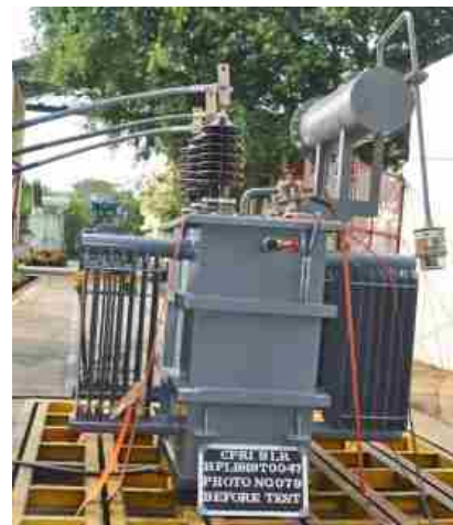
Ability to withstand the dynamic effects of short circuit tests on 315 kVA, 33/0.433 kV, Three phase transformer carried out at High Power Laboratory, CPRI, Bangalore, for M/s. OMAN Industry Transformers & Switchgear, Sultanate of OMAN
