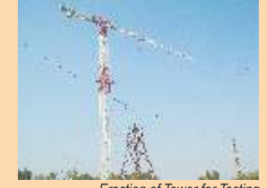
Erection of Tower for Testing
