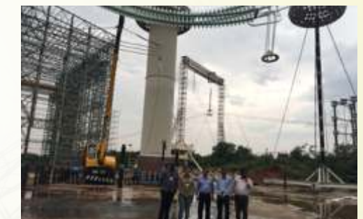
Engineers from M/s. KETRACO, Kenya and M/s. Tag Corporation, Chennai along with Officers of UHVRL
