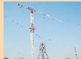
Erection of Tower for Testing
