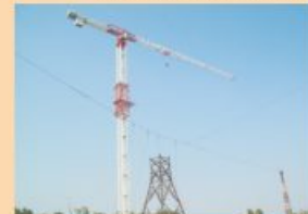
Erection of Tower for Testing
