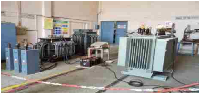
Temperature rise test, Sound Level measurement in no load & full load conditions were conducted on the transformer of M/s SGB Malaysia Compact substation as per cl. 6.1, 6.5 of IEC 62271-202, 2014. The tests were conducted in STL, CPRI, Bhopal.
