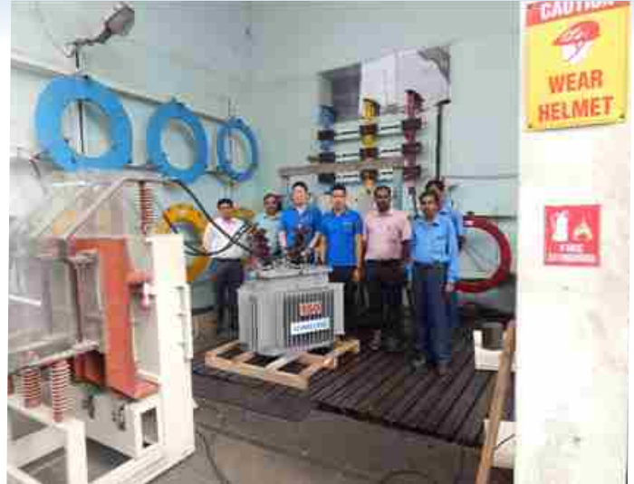
Visit of Mr. Kornchan Jeeyachok & Mr. Kittipong Pradidkaew from M/s. Precise Electric Manufacturing Co. Ltd., Thailand for witnessing the Ability to withstand the dynamic effects of short circuit test & Temperature-rise tests carried out on 160kVA 22/0.400kV & 160kVA 33/0.400kV Three Phase Distribution Transformers for M/s. Precise Electric Manufacturing Co. Ltd., Thailand
