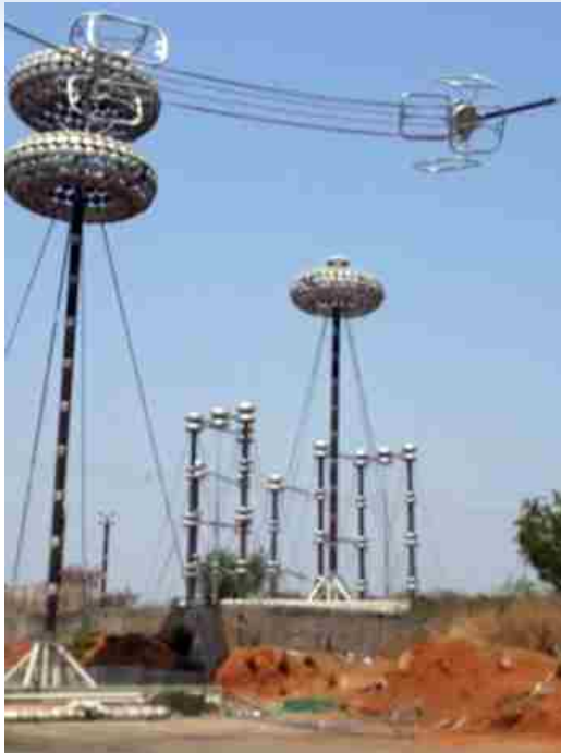
DC corona test on \pm 800 kV HVDC ACSR Hexagonal Lapwing Conductor Bundle for M/s. Neccan Power & Infra Ltd., Jaipur
