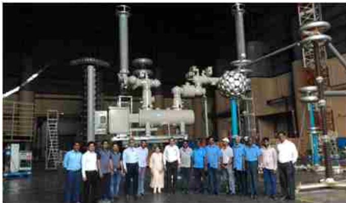
Visit of Kang dong wan, Lee Jongmin, Yun Jinwon for Dielectric and RIV tests carried out as per IEC 62271-203 on M/s. Hyosung T&D India Pvt. Ltd., Pune, make 420kV Gas Insulated Switchgear comprising of Circuit breaker and Disconnecting switches carried out at High Voltage Division, CPRI, Bangalore.
