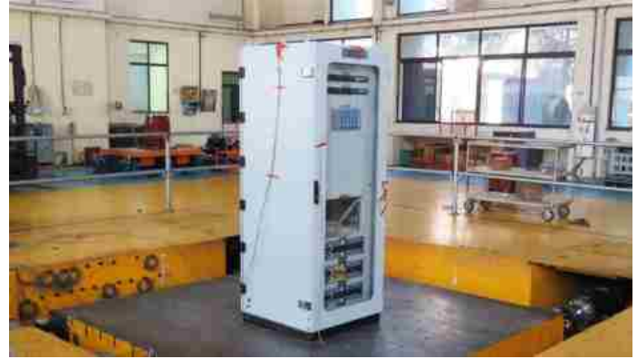
Seismic Test on Integrated Motor Control System Panel for M/s. Al-Ahleia Switchgear Co., Kuwait
