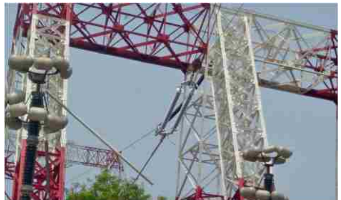
Lightning Impulse voltage withstand test and Power frequency voltage withstand test carried out on 400kV, Polymer insulator string at UHVRL-CPRI, Hyderabad for M/s. Deccan Enterprises Limited, Hyderabad
