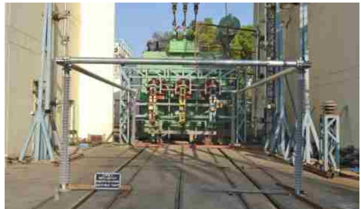
Short-time withstand current test on 220 kV rated substation post insulator for M/s. Deccan Enterprises Ltd., Hyderabad
