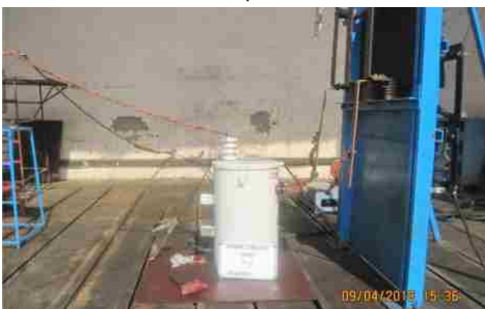
37.5 kVA, 6.35 kV/240V Single phase transformer of M/s Confidence electric Bangladesh, undergoing short circuit test in Station1, STDS, Bhopal
