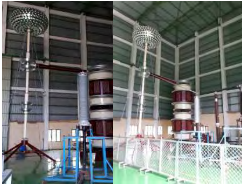
132 kV Cable test in progress
