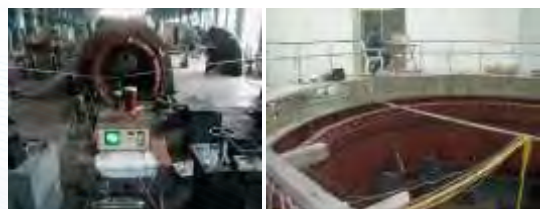
Partial Discharge test on 110 MW Turbo Generator
