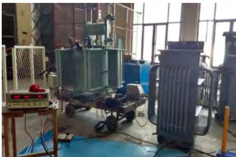
Transformer under Temperature Rise Test
