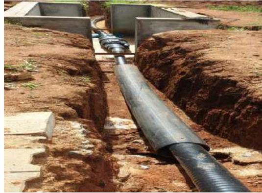
Cable laid through HDPE Pipe
