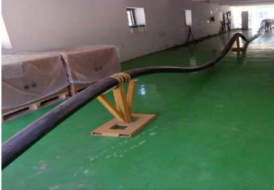
Cable in tunnel with snaking arrangement
