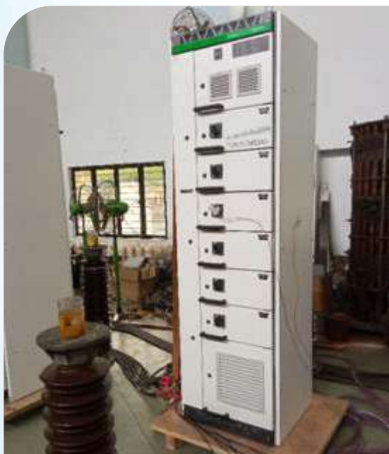
A view of the tested 3Ø, 415 V, 534 kVAR, PFC Panel
